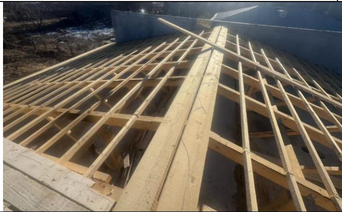
Roof construction works(Vardanashen MA)/ Kankarshin LLC and Art Plast LLC/
