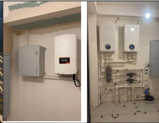
Installation of heating boilers (Akhurik MA)/ Lenchanshin LLC/
